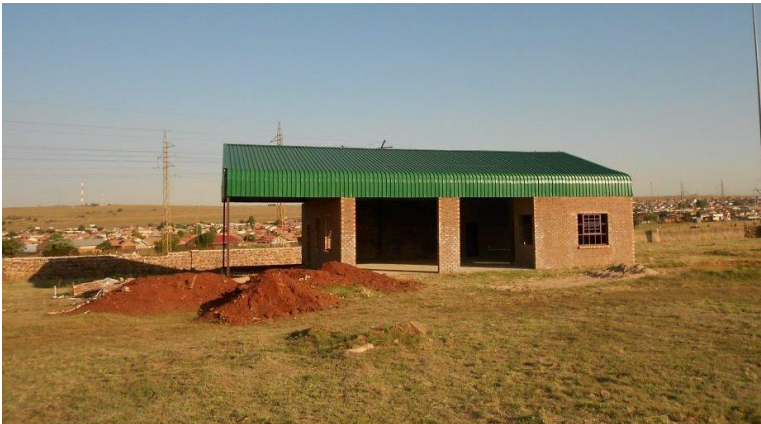
Job Training Center under construction
