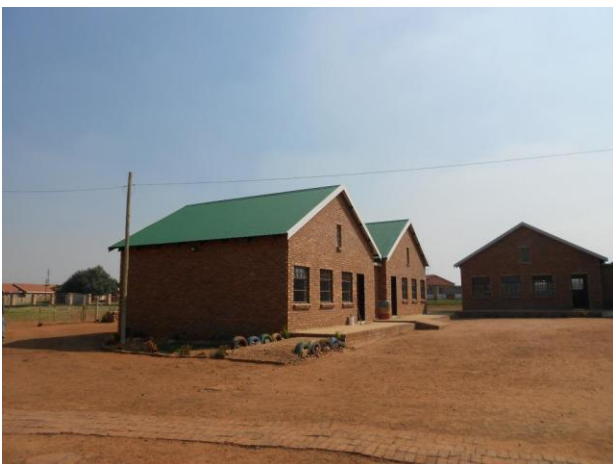
Newly built classrooms at St. Peter Christian College
